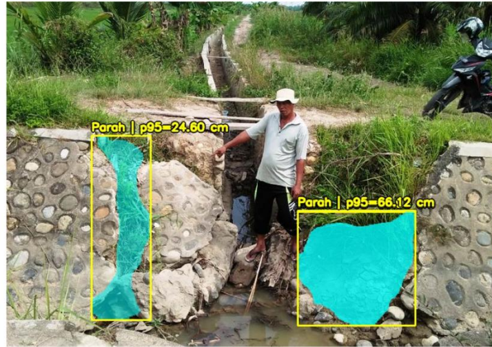
Figure 7. Qualitative mask visualization for canal damage; severity text and centimeter values in the prototype overlay are uncalibrated interface outputs and were not analyzed as study measurements
