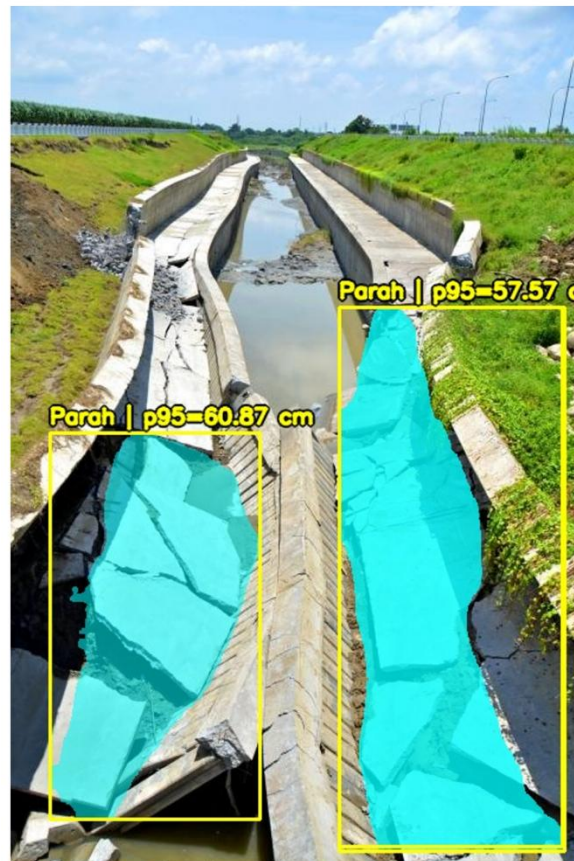
Figure 8. Qualitative mask visualization for large damaged regions; centimeter values in the prototype overlay are uncalibrated and should not be interpreted as validated physical measurements
